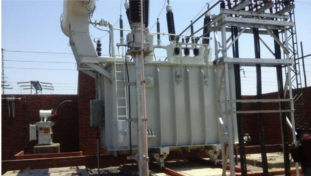
*The 20 MVA substation at Mpopoma Substation installed and commissioned on 12 November 2015*
