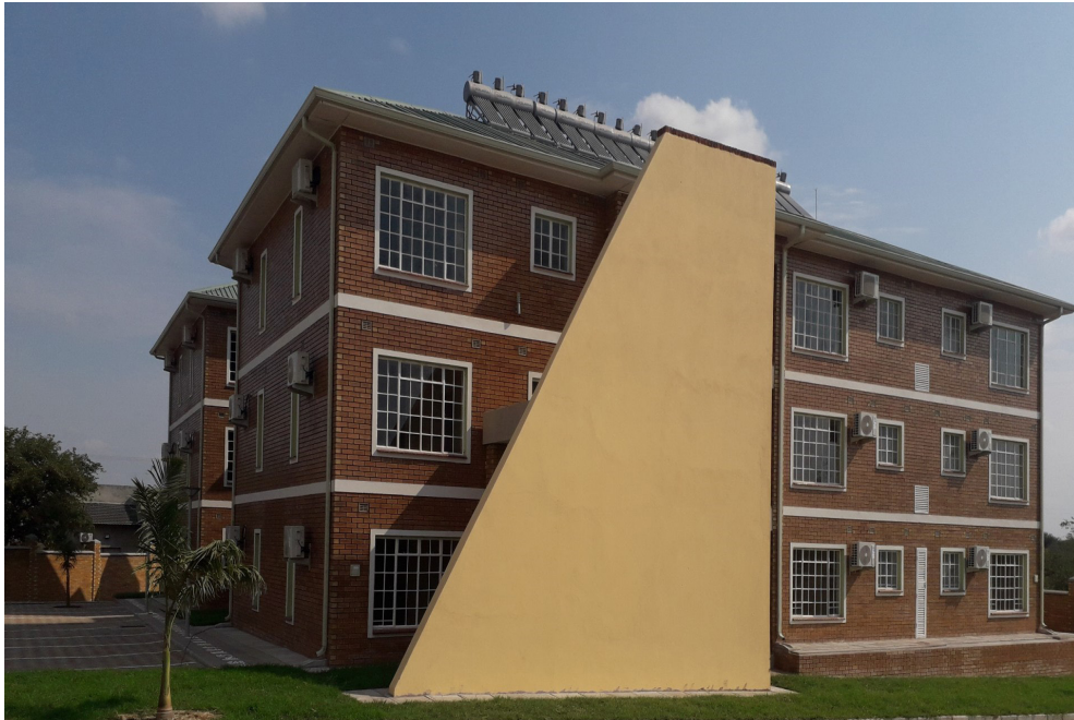
Figure 9: New Staff Housing Units at Beitbridge Border Post
